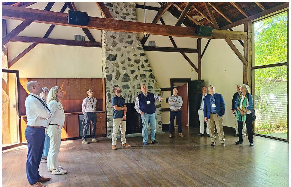
The tour stops in the barn to reflect on the visible original skip decking retained by the 1950's renovation and to discuss repairs and restoration.
